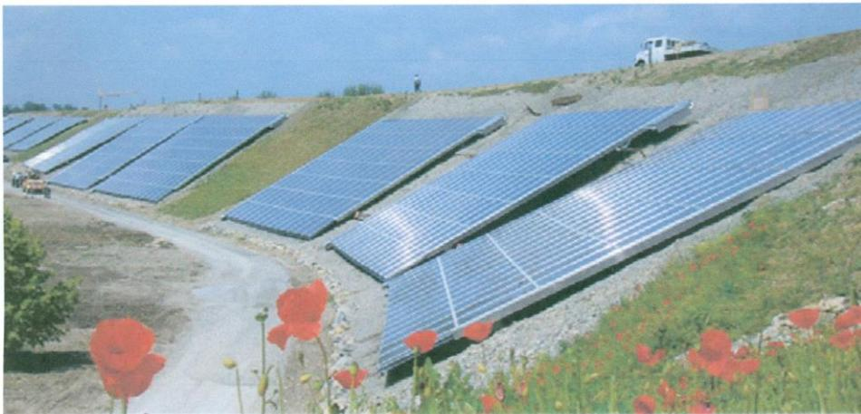
**Fig. 2-34:** Solar Collectors on a noise protection wall in Crailsheim
